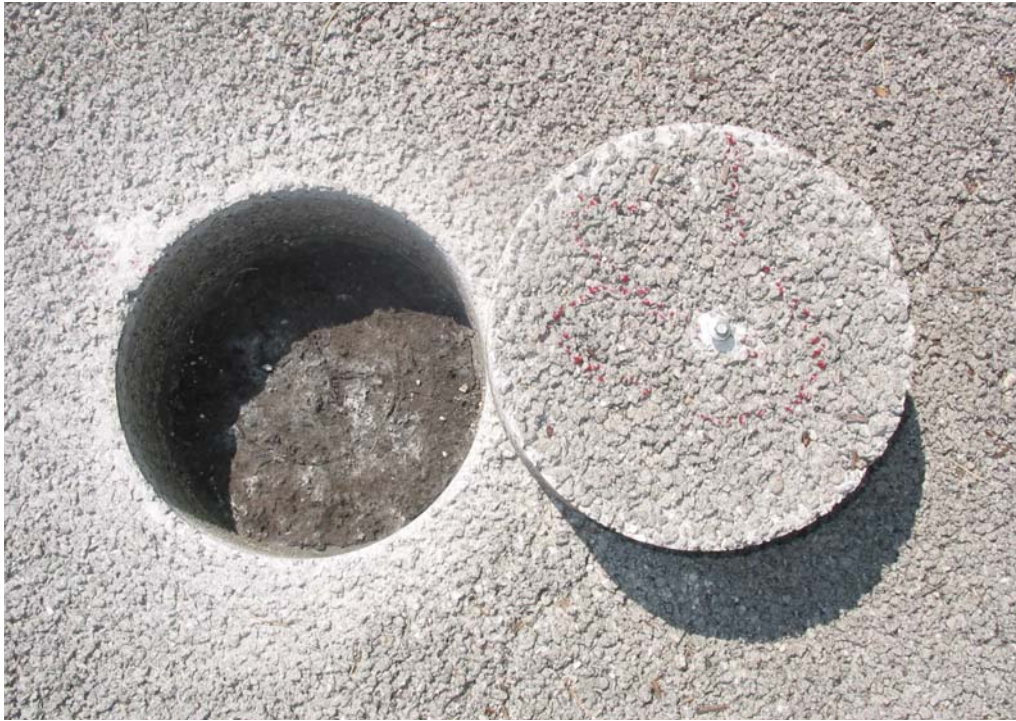
Figure 8: Pervious Concrete Pavement Core
