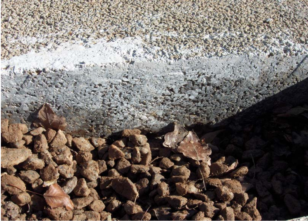
Figure 32: Cleveland Park Parking Lot Reservoir
