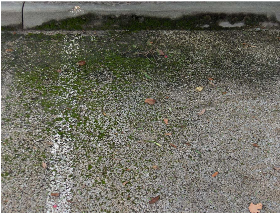
Figure 24: FCP&A Parking Lot
