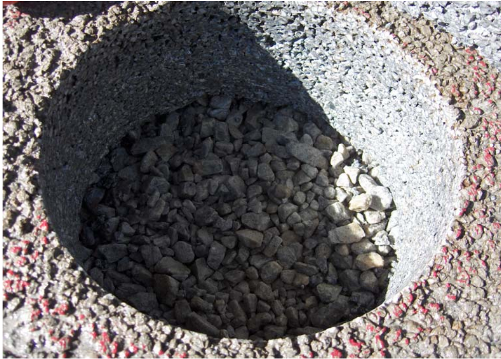
Figure 27: Southface Institute Gravel Subbase
