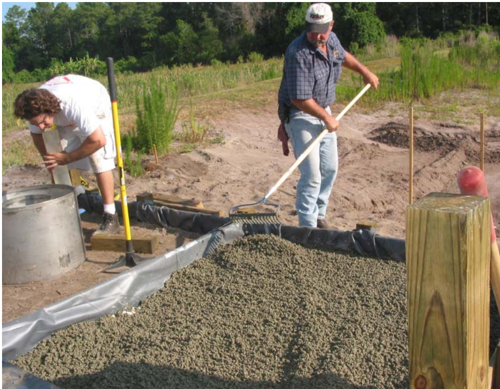
Figure 3: Stormwater Academy Porous Concrete Test Cell Installation
