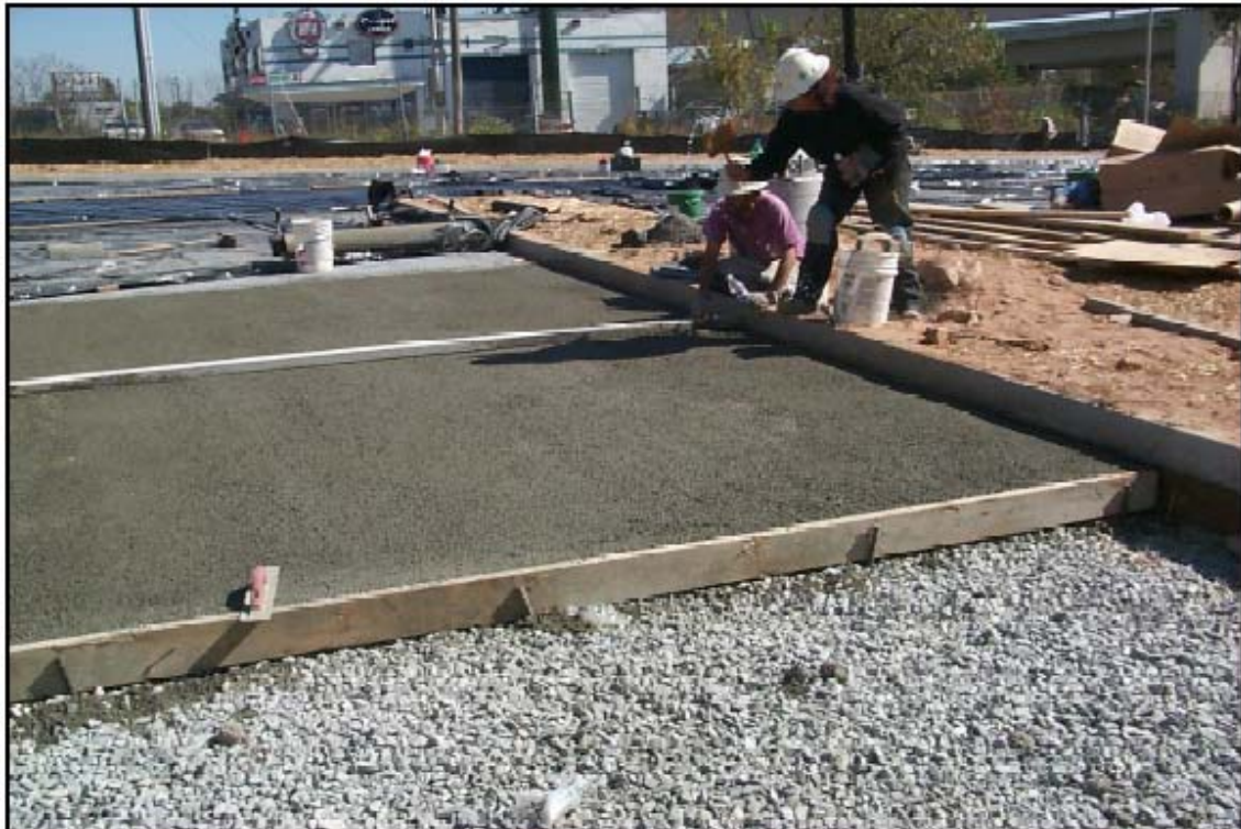
Figure 2: Typical Porous Concrete Installation
