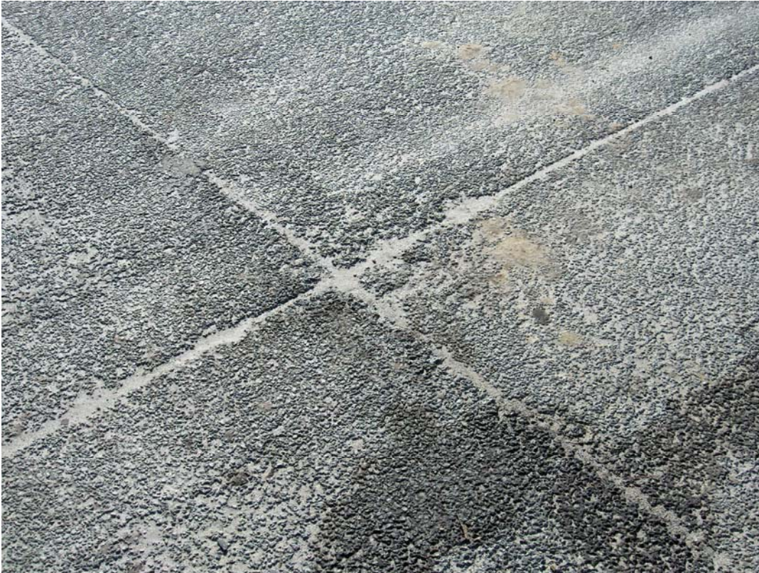
Figure 35: Effingham County Landfill Pervious Pavement
