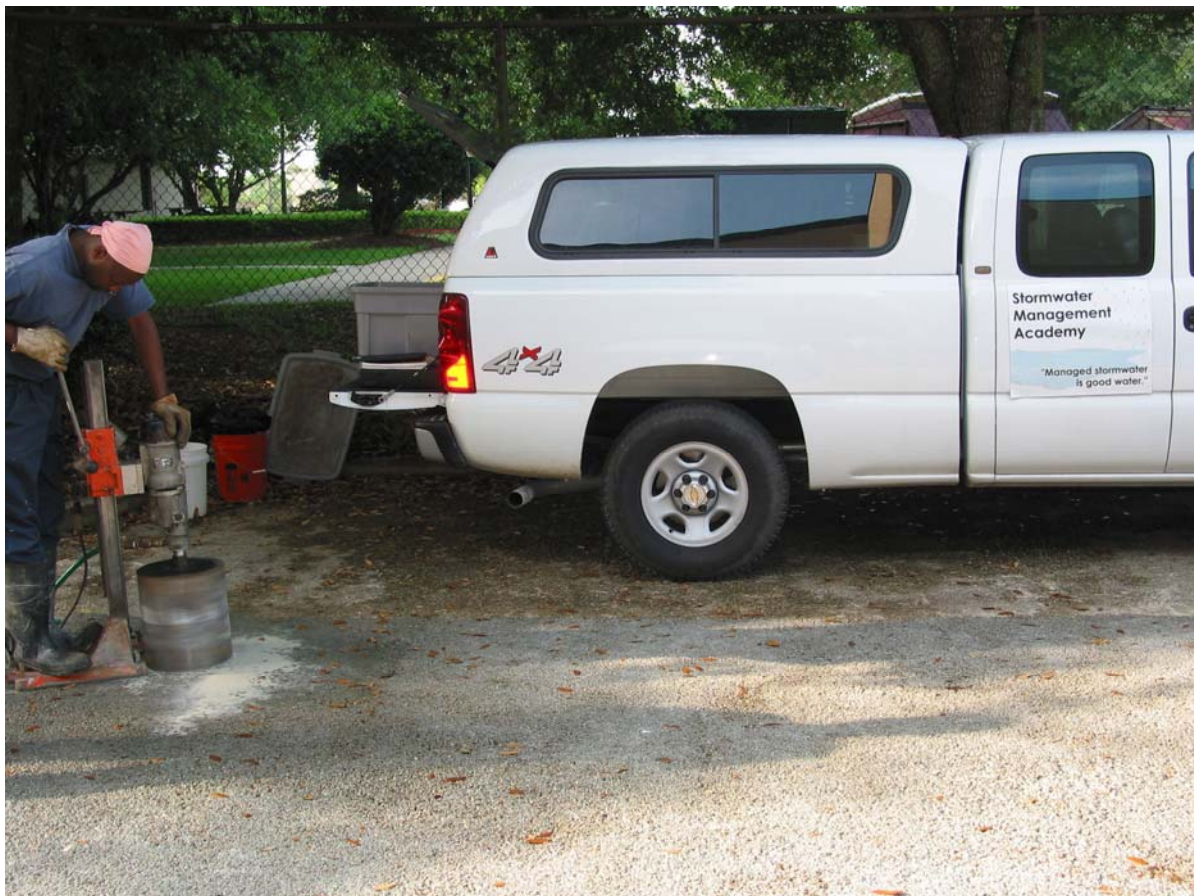
Figure 22: FDEP Parking Lot Core Test
