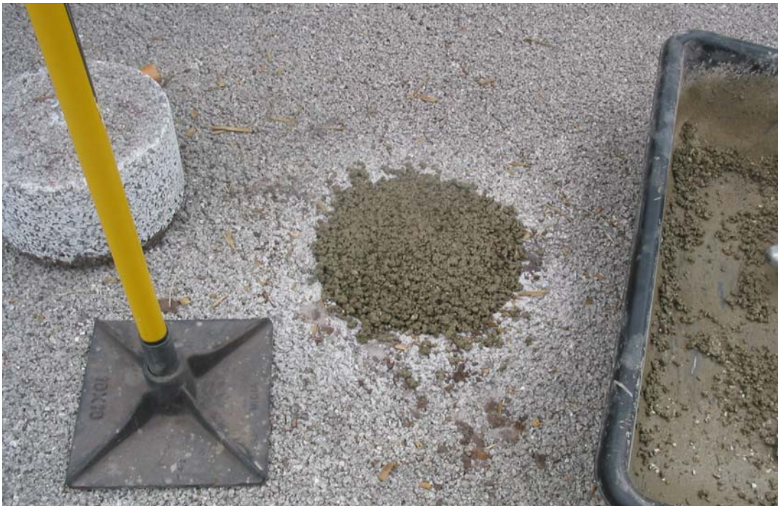
Figure 11: Repair of Concrete Core Area
