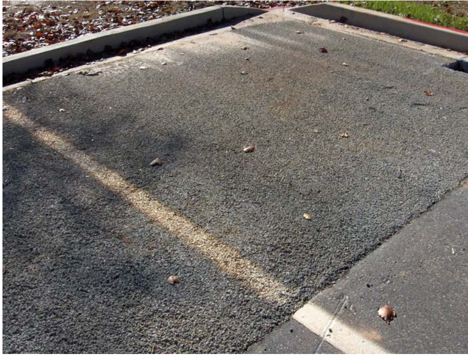
Figure 31: Cleveland Park Parking Lot Pavement
