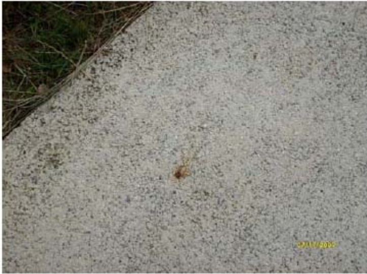
Figure 13: Surface sealed by wet mixture or over compaction
