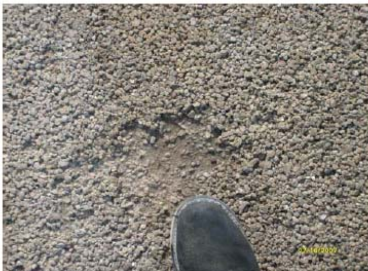
Figure 3: Surface raveling (observed at Charter School, Gary, Indiana)
