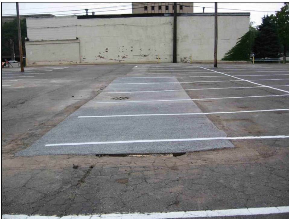
Figure 19: CSU Parking Lot D Demonstration Project
