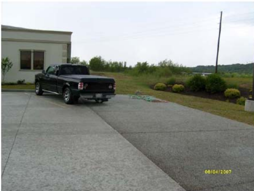
Figure 23: Harrison Concrete Plant, Harrison, Ohio
