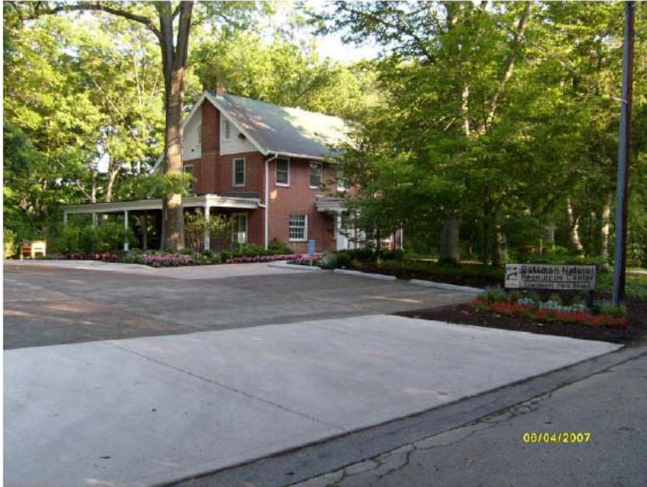
Figure 18: Bettman Natural Resource Center parking lot, Cincinnati, Ohio
