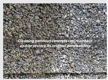
Deep cleaning/unclogging is best accomplished by simultaneous pressure washing and vacuuming. Several equipment manufacturers have developed pressure washing/vacuum systems that have proven to rehabilitate the pore structure of pervious pavement. For best results, follow the equipment manufacturer's recommendations. As with the periodic maintenance procedures, when cleaning/unclogging is performed, a maintenance log should be completed and filed with the owner/property manager.
