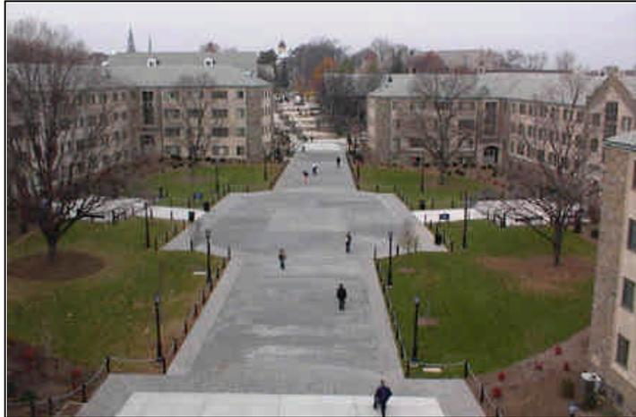
outfitted with three infiltration beds overlain with pervious concrete. The site originally had a conventional storm sewer system which channeled runoff directly to the headwaters of Mill Creek, a high-priority stream on Pennsylvania's Clean Water Act (303d) List. Usage of the site consists primarily of pedestrian traffic with some light automobile traffic. The site also serves as a stormwater research facility.
